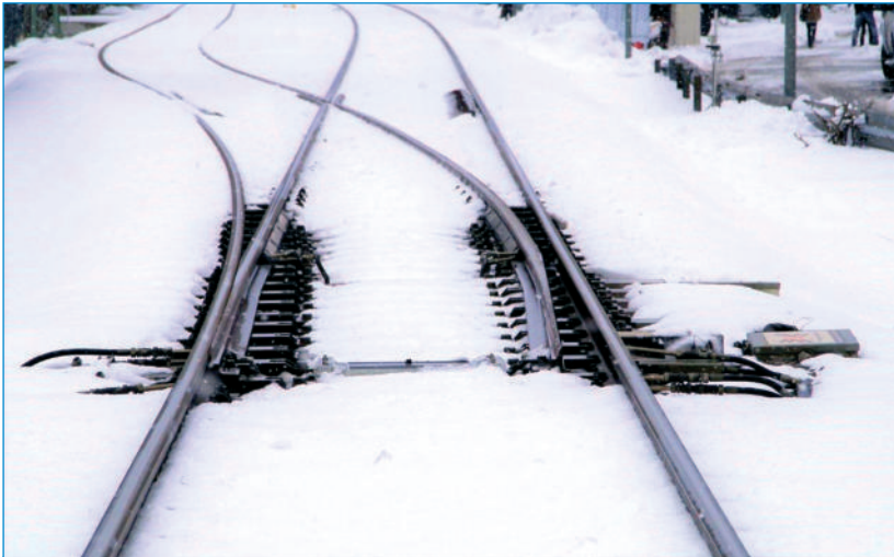
Geothermally heated railway tracks. Copyright: GRETA Project ■
