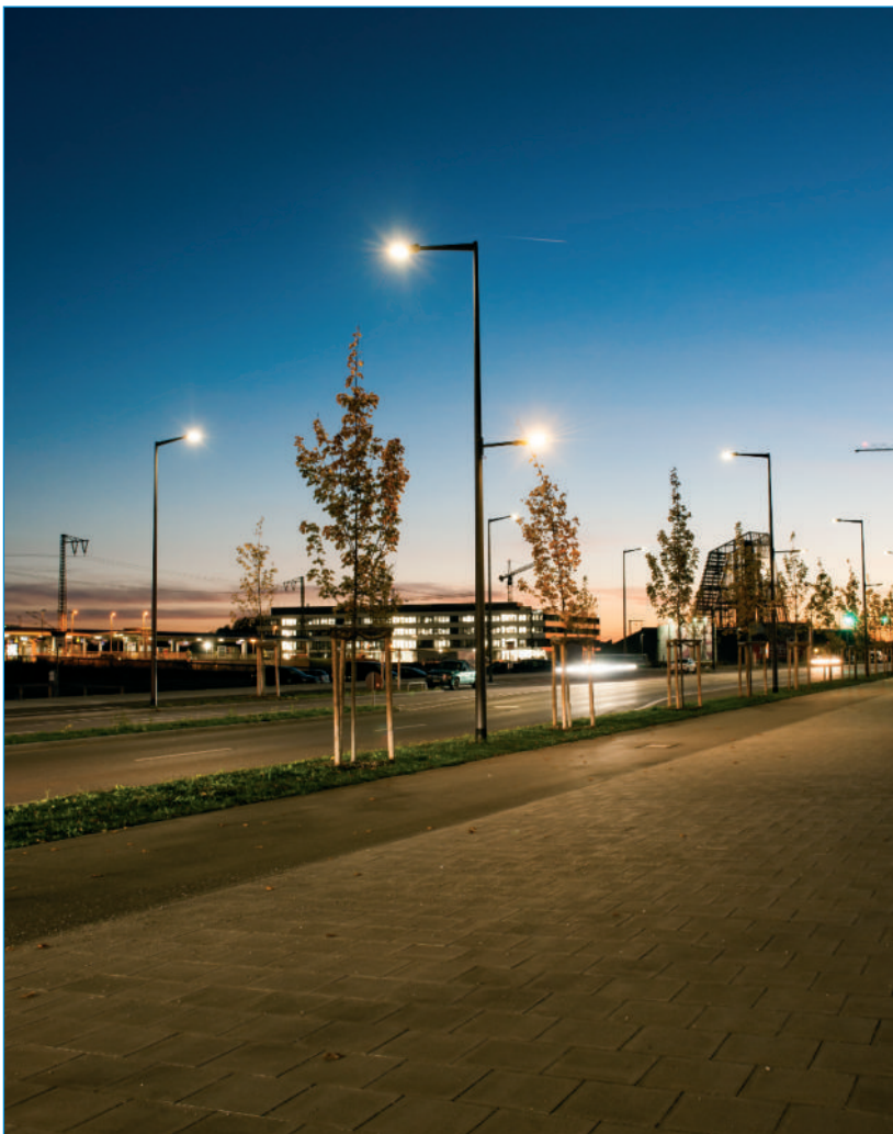
Project area/subject street lamps. Copyright: Dominik Parzinger ■
