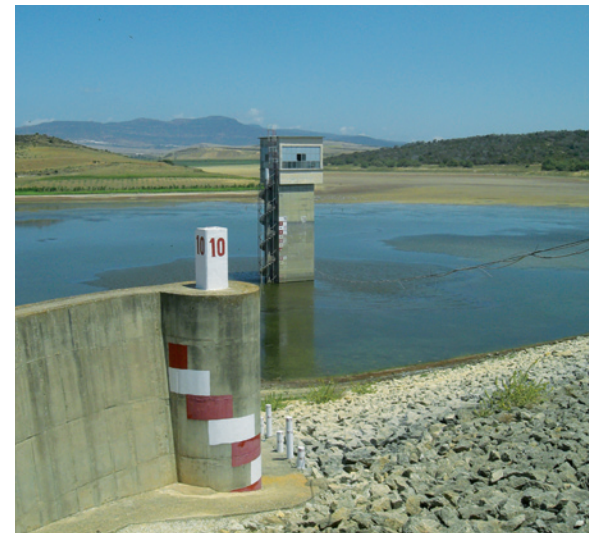
June 2010: Chiba Dam, Tunisia
